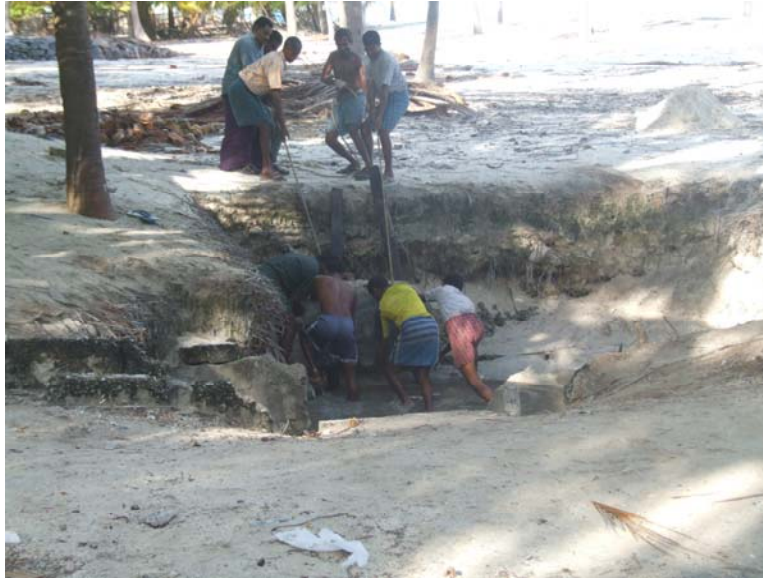
Pond construction under MGNREGS at Agatti Island
