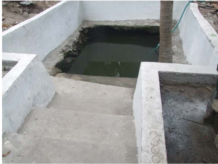
Renovation of Pond under MGNREGA at Kalpeni Island
