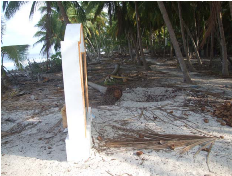
Area demarcated for ring road construction Scope for rural connectivity under MGNREGS
