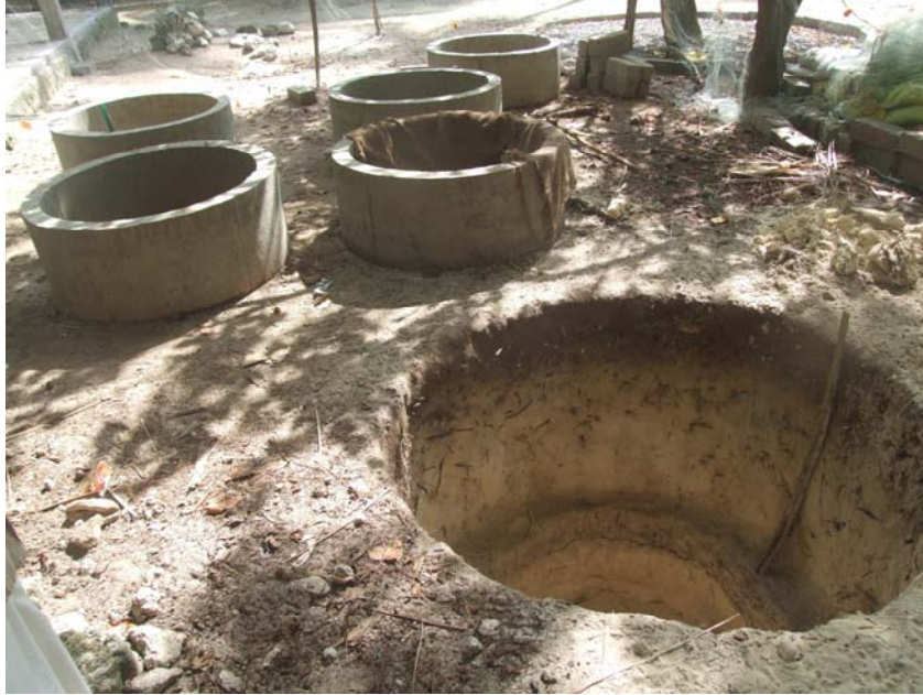
Construction of well under MGNRES at Agatti Island
