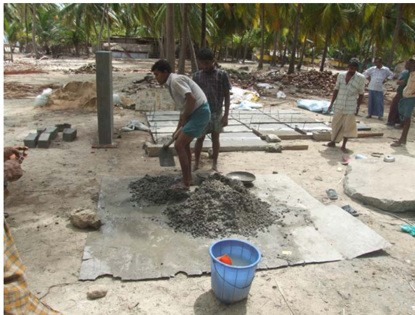
Pond construction under MGNREGS at Agatti Island
