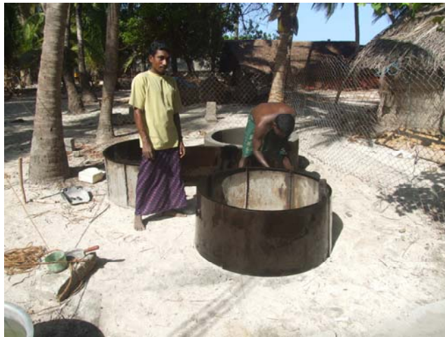
Construction of ring for wells under MGNREGS at Agatti Island
